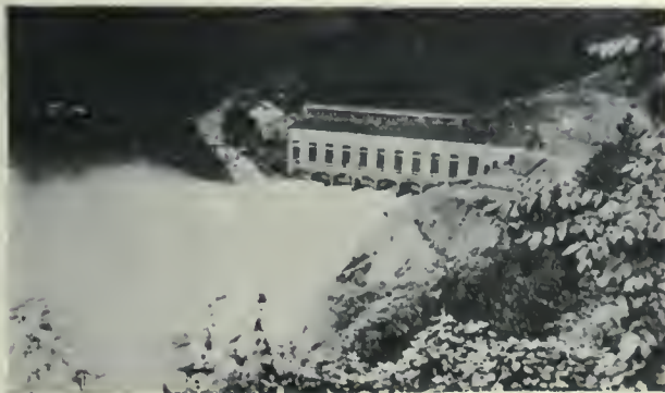
Relief valves of 16-8000 h.p. wheels discharging under head of 1500 ft.
